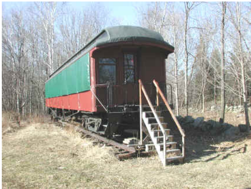
The new steps, side curtains and a corner post in need.
